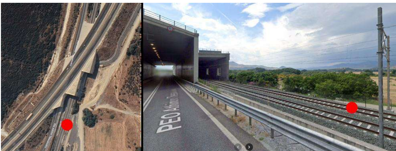
Figure 3. Photos of the tunnels on the site of the accident (left, satellite – right, from the road beside)
